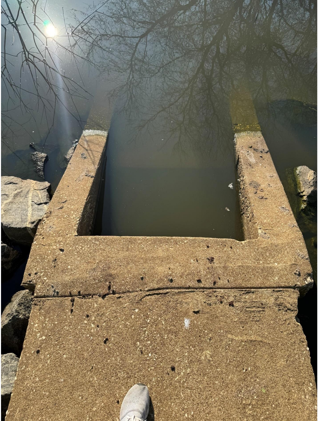
Photograph 8: Downstream Outlet of Discharge Pipe through Dove Pond Dam
